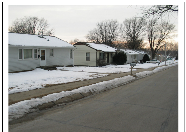
Single family units similar to these have a good residential scale.
